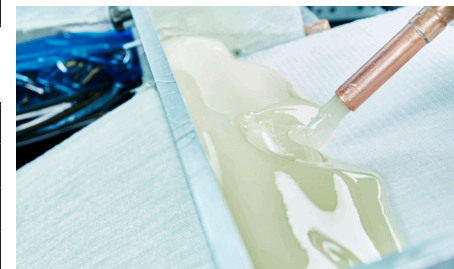
Impregnation with UP resin
